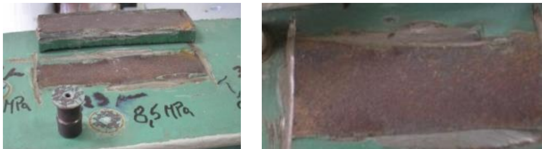
Figure 15. Panel No. 7 (C condition) – appearance of the angle bar after seasoning, with a flat bar cut off (left), enlargement of the bottom of the flat bar (right)
