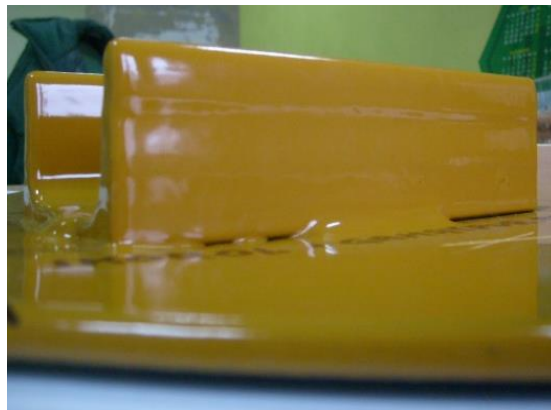
Figure 8. Panel No. 3 (BSa2.5 condition) – the appearance of a welded C-profile, the lack of contact of both planes is visible, despite the application of paint with an average thickness of 1302 \mu\text{m}
